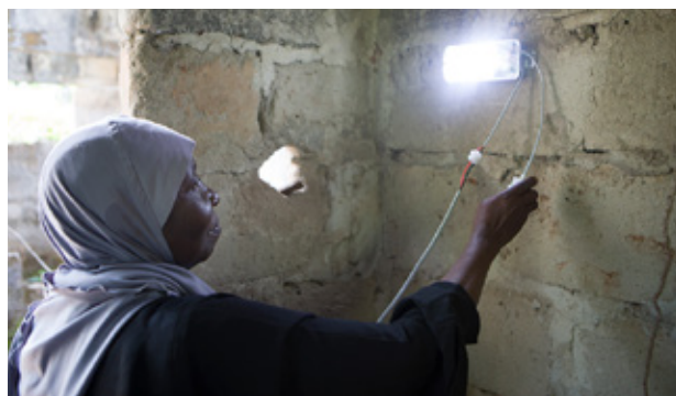
Zanzibaris Engineer, Amina has installed 100 solar home lighting systems.
